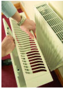
Step 7/8. Once the radiator has been fitted securely to the wall use a key to separate the front cover from its casing. Place the appropriate LST cover over the top and mark drilling holes.
