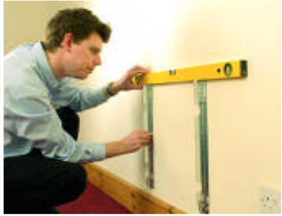
Step 4. Ensure the brackets are level.
