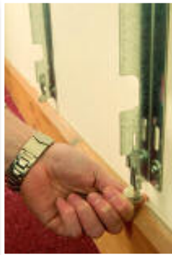
Step 5. Insert the plastic grommets onto the brackets (these minimise expansion and contraction noise). Pull down the spring loaded part of the bracket, and push it back to locate it in its lower position.
