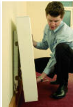
Step 6. Hook the radiator lugs on to the tops of the brackets. Return the spring loaded part of the bracket to its original position, thereby securing the bottom of the radiator in its final position.
