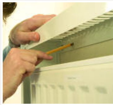
Step 7/8. Once the radiator has been fitted securely to the wall use a key to separate the front cover from its casing. Place the appropriate LST cover over the top and mark drilling holes.
