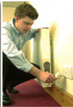
Step 6. Hook the radiator lugs on to the tops of the brackets. Return the spring loaded part of the bracket to its original position, thereby securing the bottom of the radiator in its final position.
