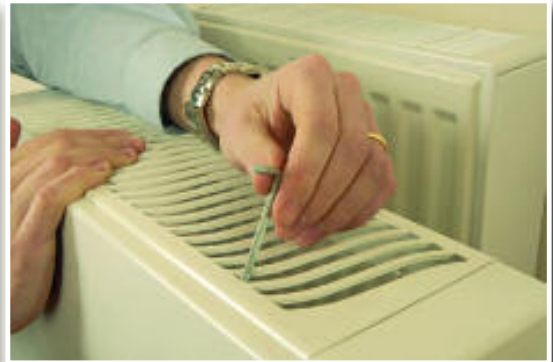
Step 7/8. Once the radiator has been fitted securely to the wall use a key to separate the front cover from its casing. Place the appropriate LST cover over the top and mark drilling holes.
